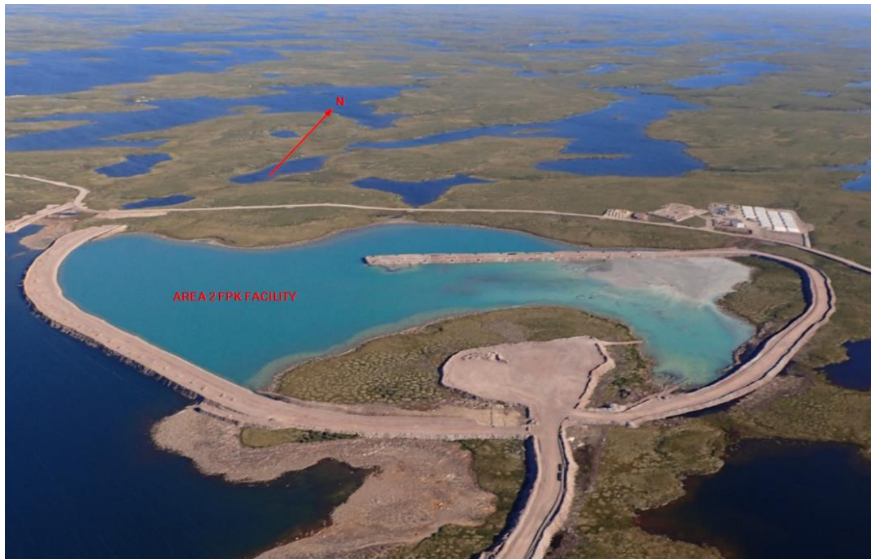
Figure 17-4: Area 2 Fine Processed Kimberlite Facility Q3 2017
