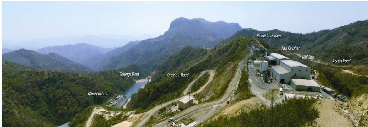
Figure 18-1 Photograph Looking Southwest Showing Access & Haul Roads, Power Line, Mine & Mill Sites & Previous Tailings Dam
