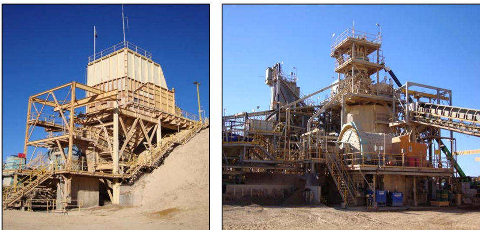
Figure 34: Paroo Station crushing and grinding sections
