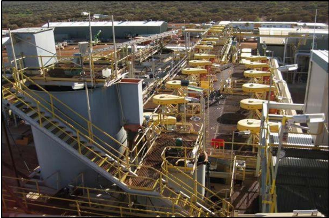
Figure 35: Paroo Station flotation section
