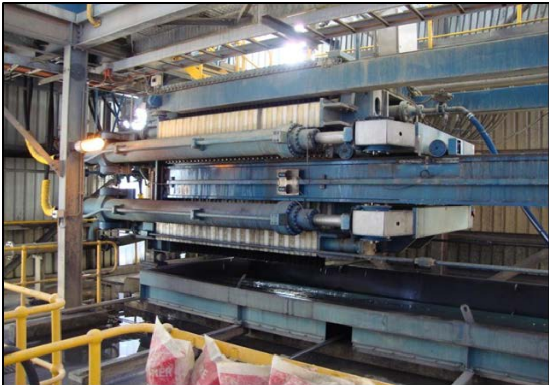
Figure 36: Paroo Station lead concentrate filter
