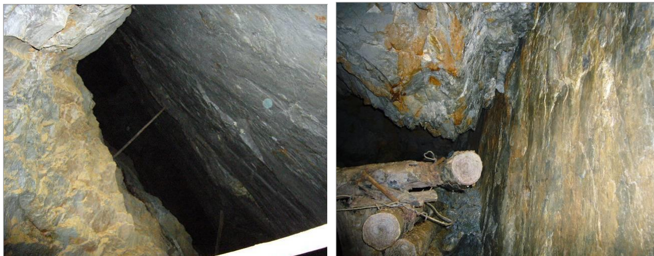
a) Vertical and smooth fault plane of NE vein V10 in an open stope of Tunnel ML5.
