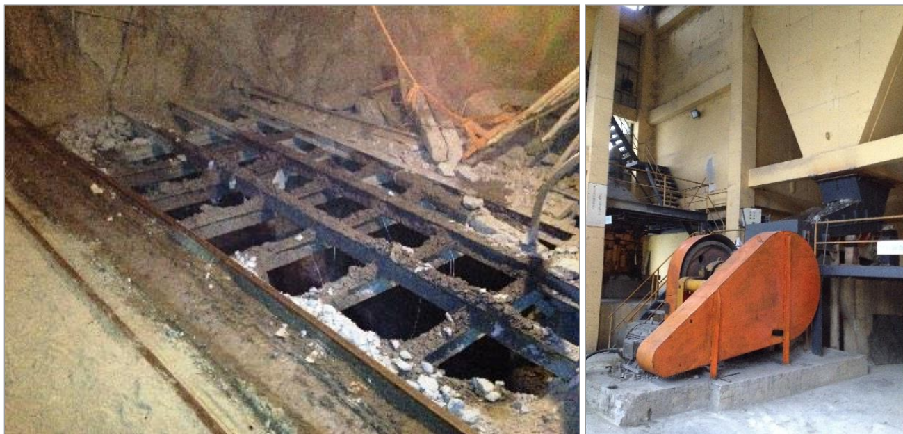
Figure 17.3 Surface grizzly feed to ROM ore bin
